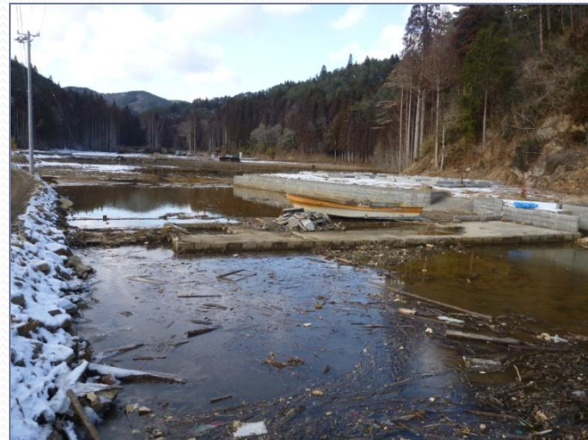
Investigating the potential for reclamation of wetlands for subsided land at Karakuwa, Kesenuma City
