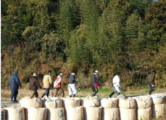
Sandbags were piled as a temporary levee
