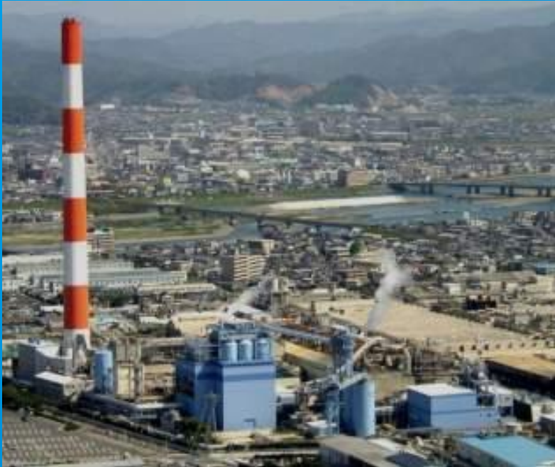
Four thermal power plants
