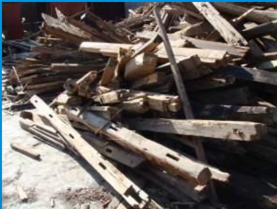
建築廃材 Wood material from construction waste
